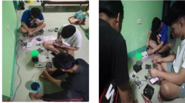
Checking of Wires
